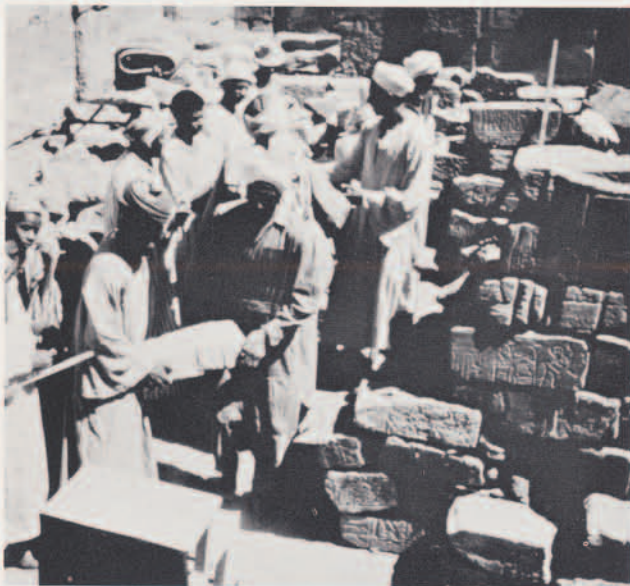
Stacking blocks from the demolished Akhenaten Temple at Karnak.
