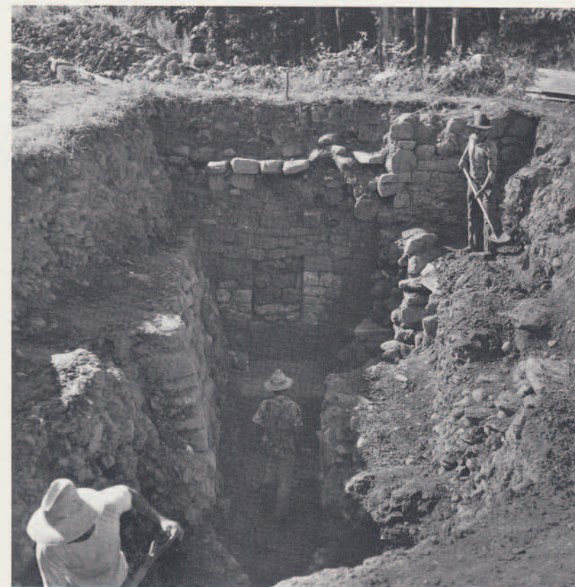
14 Excavation into the room of a structure completely filled and buried by Construction Stage 1.
