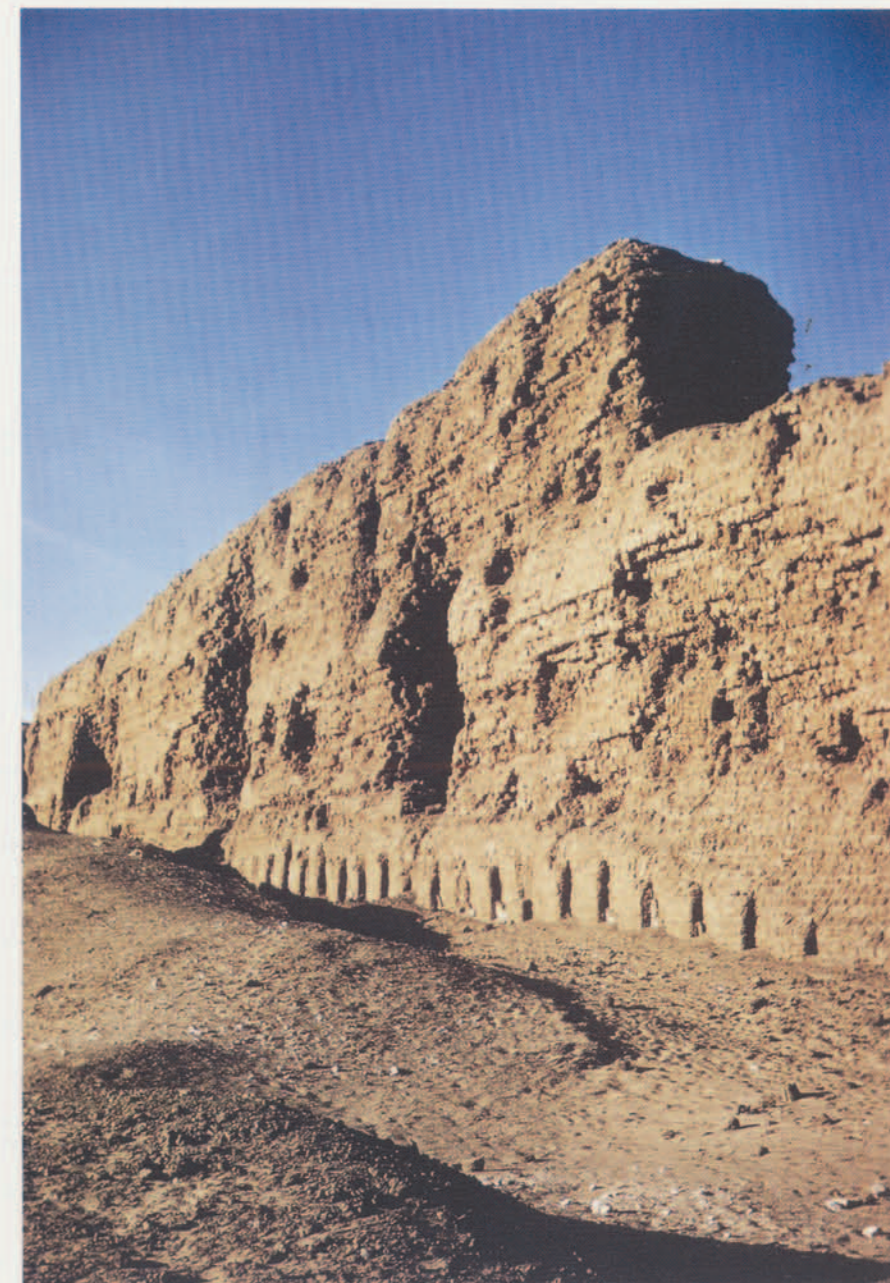
17 The east wall of the Shunet el Zebib.
