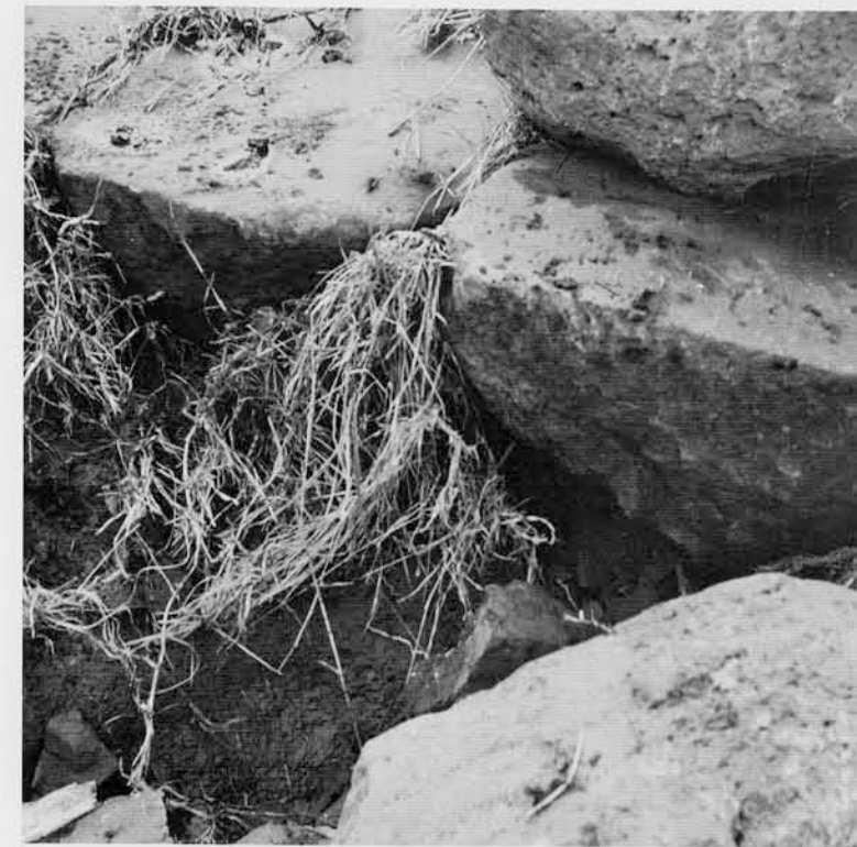
Details of Roman paving stones. The round stone has been cut to form the edge of the road and would have been fitted against the curbing stones.
