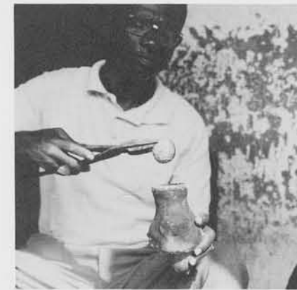
6. Pouring gold into the mold
