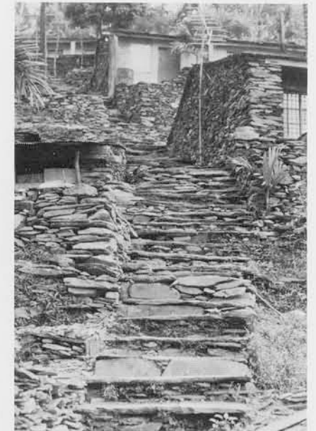
9 Slate construction of Budai village.
