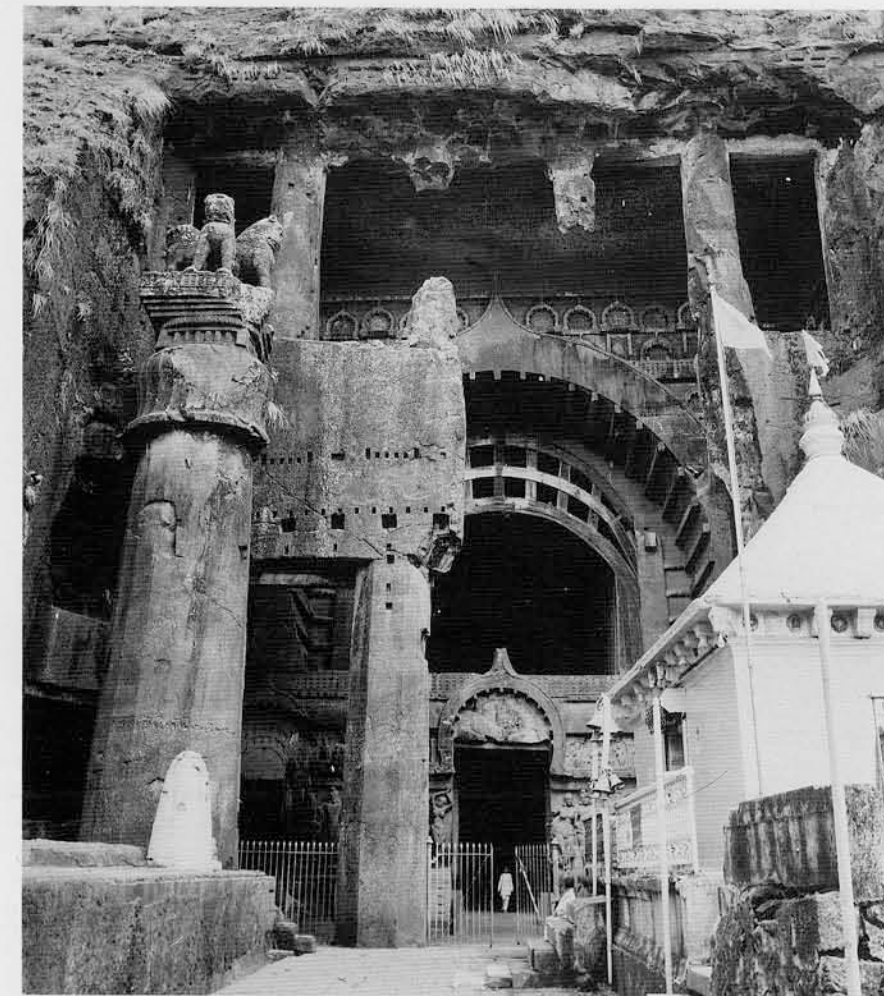
5 Entrance to a chapel at Karle, showing the arched facade with intact wooden ribbing under the arch. The holes visible above the pillars in front of the arch also supported a wooden structure. (Photo courtesy of AIIS)
