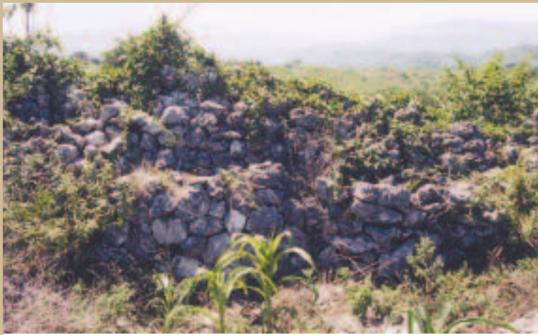
The defensive wall at the site of Tzulublaj has a parapet halfway up its internal face which allowed defenders to man the walls without exposing their bodies to attackers.
