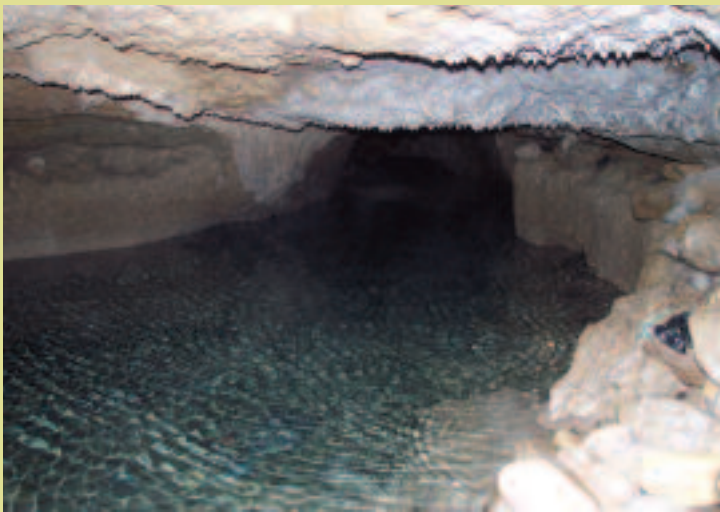
The interior of a subterranean irrigation channel ( qanat ) at Sefid Ab used to distribute water collected near the Karkas Mountains to the arid plain around Kashan.
