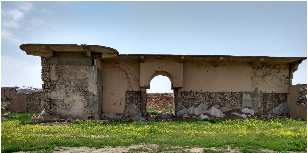
Image: The remains of the reconstructed entrance to the Palace of Ashurnasirpal II. ISIS detonated explosives in this building in 2015. To protect the original fragments, they are now covered with geotextile. Photo: Penn Museum. Available for download here .
