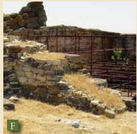
Installation of vegetative “soft” caps on north gate complex: (a) existing concrete cap prior to intervention, (b) “soft” cap protection layer, (c) capillary break layer, (d) filter layer, (e) completed “soft” caps, (f) view looking east of completed north gate “soft” wall caps, 2010.
