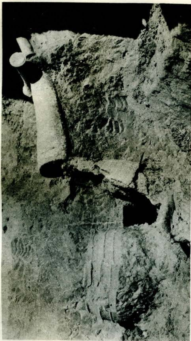
DRAIN PIPES IN THE PREHISTORIC TOWN AT UR
