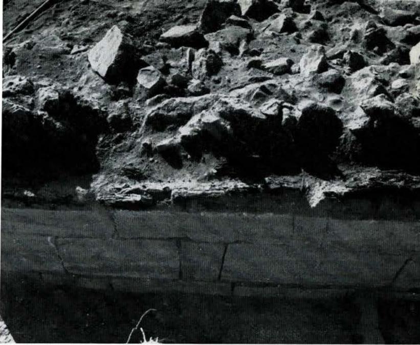
Figure 14. Wooden beams on top of the west end of the south wall of the Gate Building.
