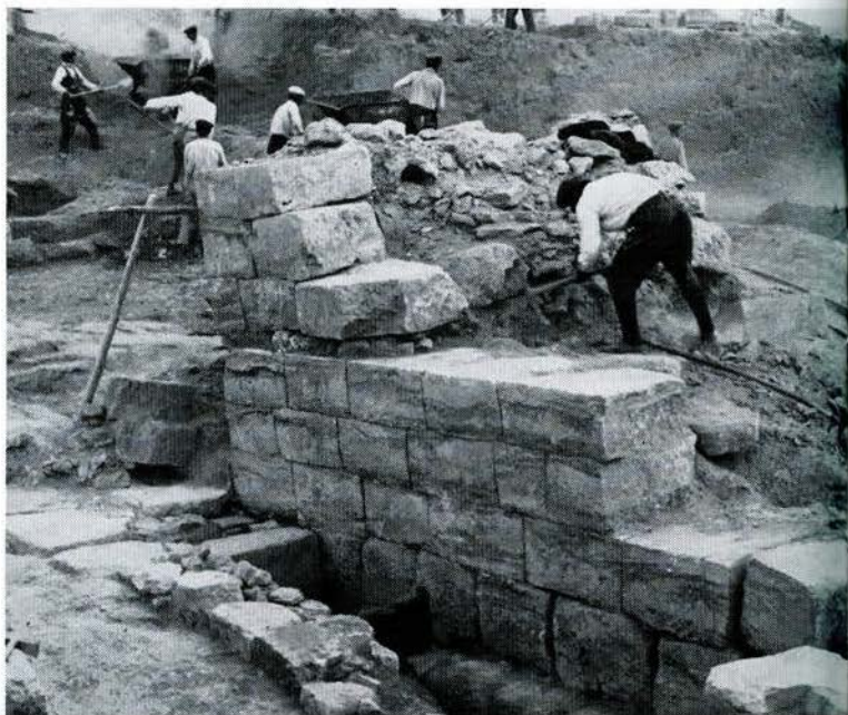
Figure 13. The south wall of the Gate Building; note the slot which once held wooden beams, between the third and fourth courses from the top.
