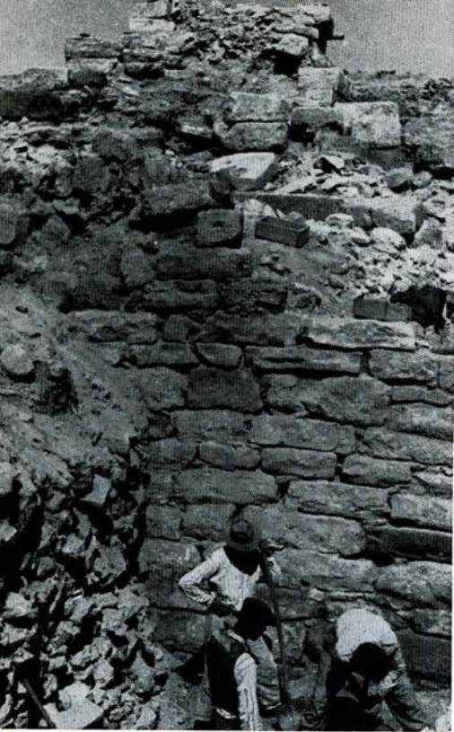
Figure 18. The outer face of the early wall beneath the Gate Building; at left, rubble foundation for the south wall of the Gate Building.
