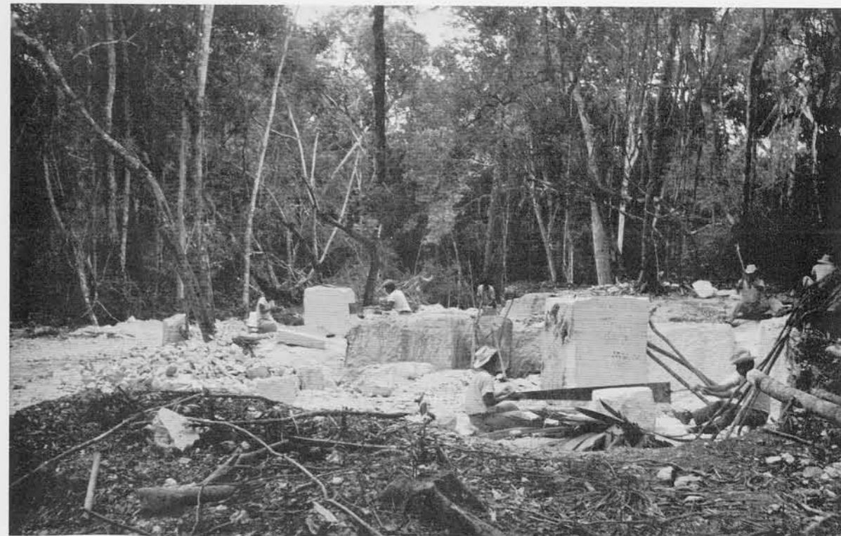
Cutting stone by handsaw in the quarry.
