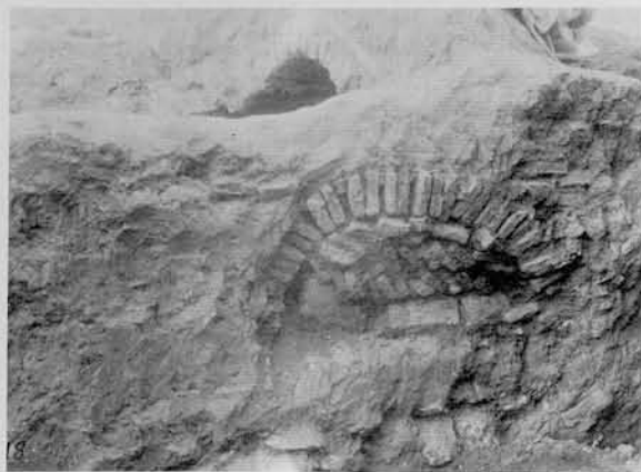
11 RT. 789: the southeast wall of the tomb-chamber from the outside showing the arched dome and door blocking of brick and stone and the collapsed vault behind.
