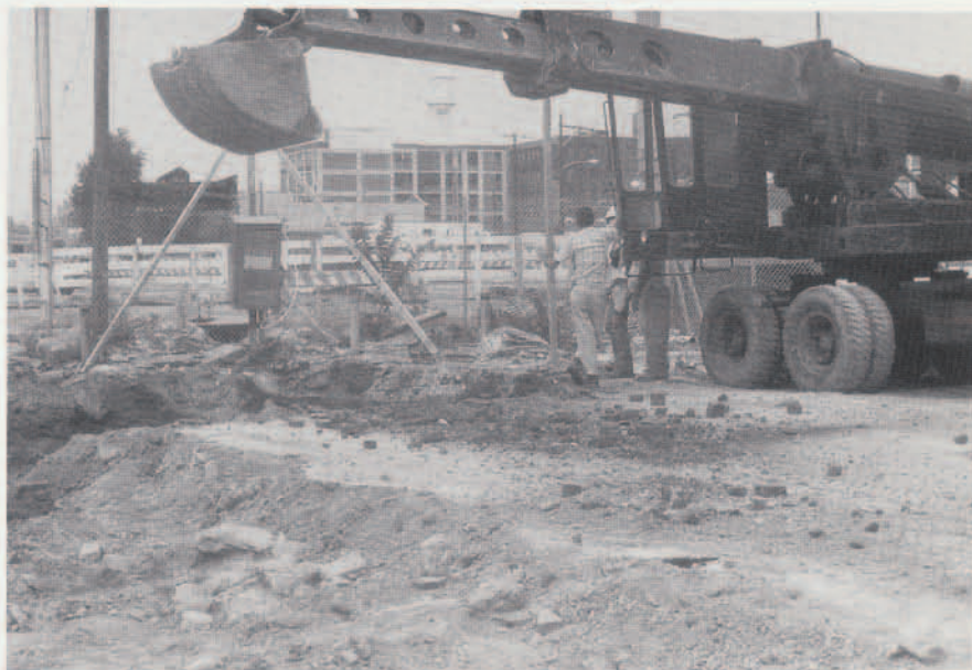
1 View of Gradall being used to clear the site.
