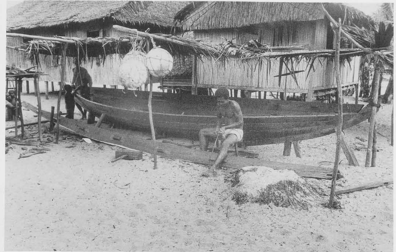
10 Building a belang prahu, Feruni.
