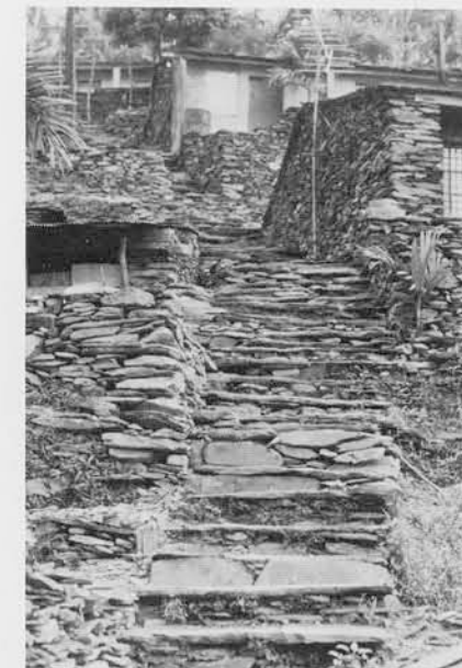
9 Slate construction of Budai village.
