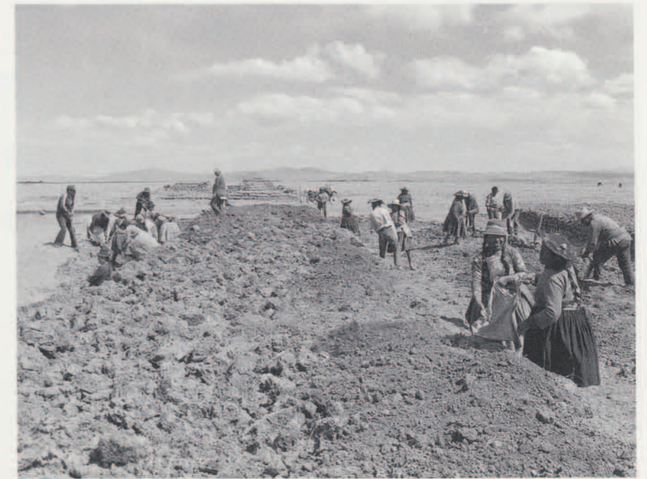
9 Community lands are cultivated today by representatives from each family household, an old Andean pattern of communal labor. Here, the final construction of a large raised field platform of the Community of Yasin in Chojñocoto, Huatta. Loose soil is tossed on the field using carrying cloths to create a convex surface over the sod blocks which make up the fill (September 1985).
