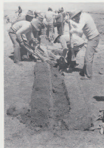
6 (above) Members of the Community of Segunda Collana using footplows to cut sod blocks from old canals for the retaining walls for rebuilding the raised field platforms in Viscachani Pampa, Huatta (October 1985).
