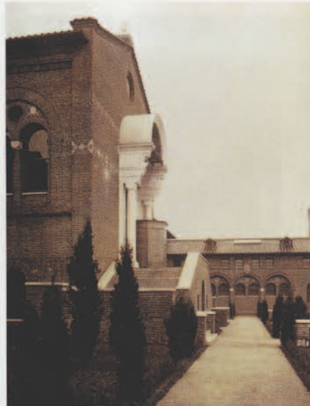
The upper courtyard of the Museum shortly after construction, ca. 1899.
