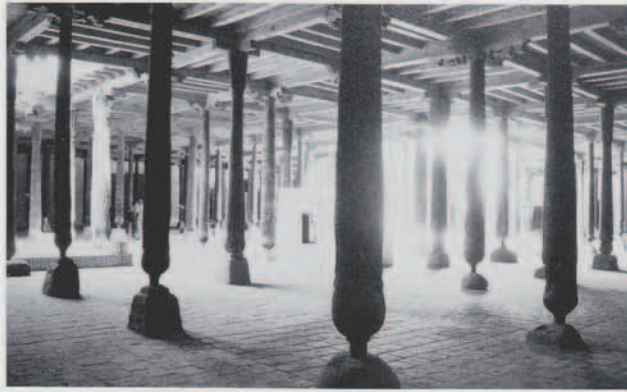
Fig. 9. Ornately carved wooden columns support the weight of a great mosque of the 19th century AD in the walled oasis center of Khiva in northern Uzbekistan. (One of these columns will be in the Ross exhibit.) H. of column ca. 3.5 m
