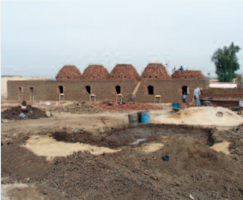
The newest wing of the dig house was constructed in 2000. Since reinforced concrete has become the preferred building material in Egyptian villages, it was a difficult task to locate masons to build the house's new domes.
