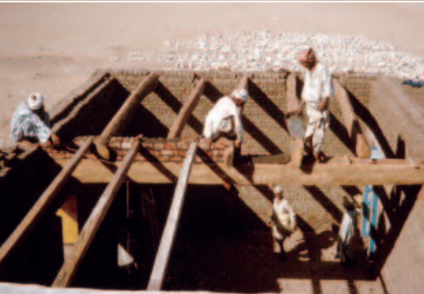
Before construction could begin in 1967, ruins of the previous structure were removed (top). Afterward, mud-brick architecture was used to construct the new dig house (middle), with wooden rafters supporting the flat roofs (bottom).
