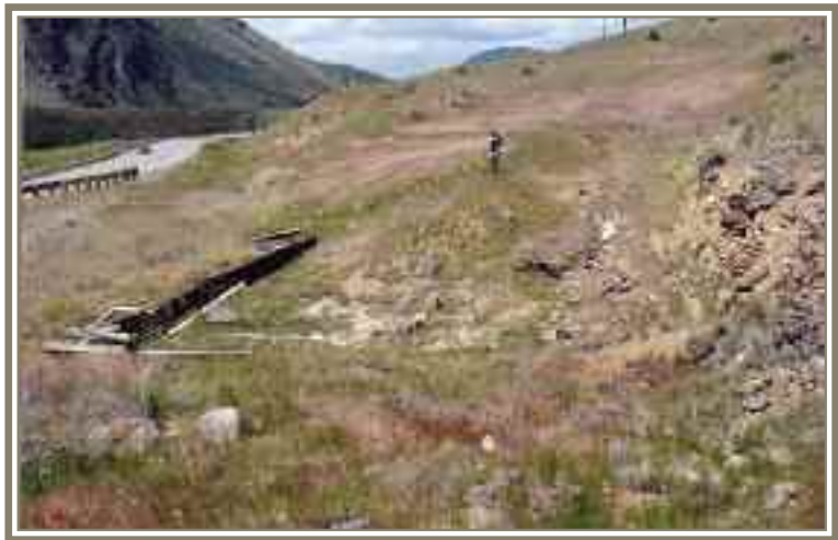
The construction of Highway 89 destroyed whatever was left of the resort. All that remains of the bathhouse are remnants of the foundation and concrete collection boxes that later diverted water from the springs to Corwin.
