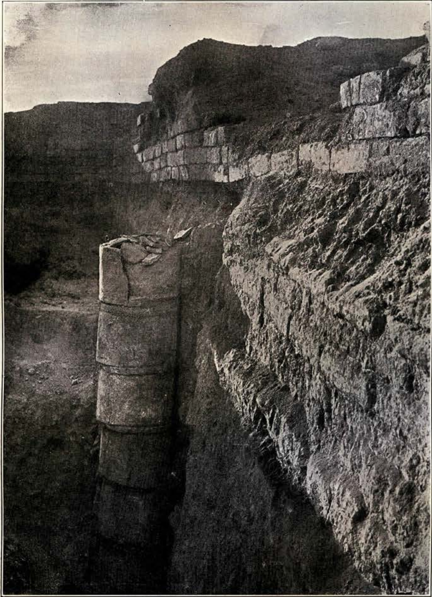
Drain pipe below the floor in the Temple of the Moon God.
